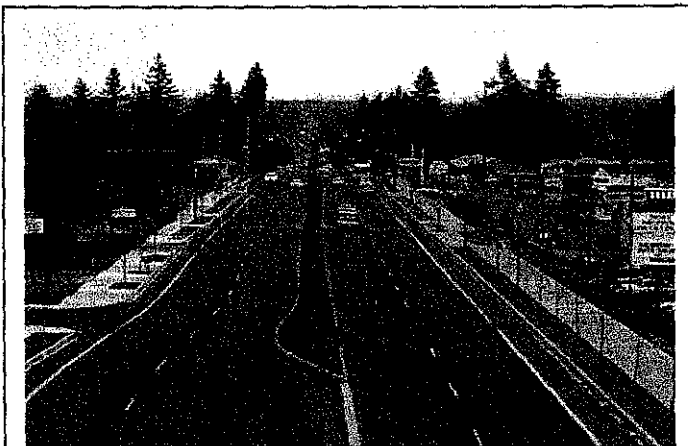
Bridgeport Way Phase I Completed Street Improvements
