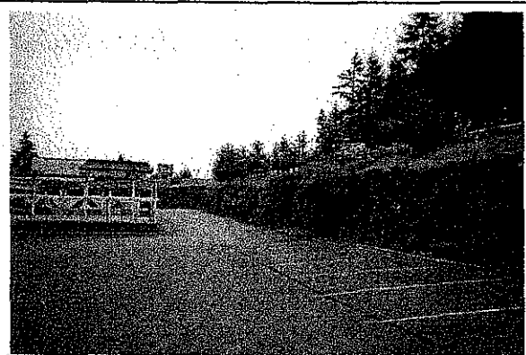
Steep Slopes along Bridgeport Way create sunken sites with poor visibility and difficult access.
