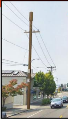
Hollow Power Pole Full Concealment
