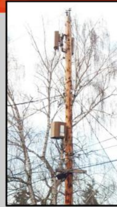
Wood Power Pole Installation in Communication Space
