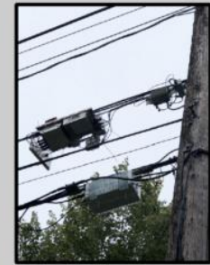
Strand Mount Attachment to Wires
